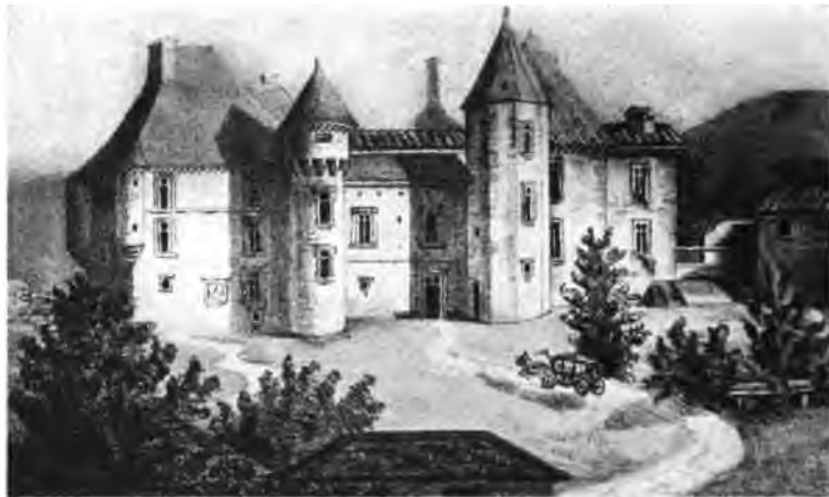
View of the Château Montaigne. The façade towards the courtyard.
