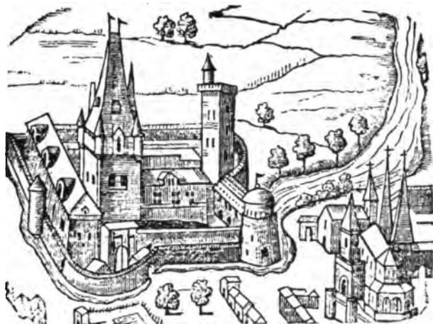
The Fort du Hâ, opposite Montaigne's house in Bordeaux
